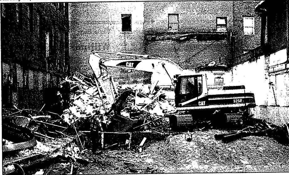
Crews remove a loading dock from a section of Riverdam Mill Monday afternoon as part of a $14.4 million project to create The Mill at Saco Falls. The section of building behind the debris will be removed to allow for better river views and easier access to the falls below. (Gillian Graham photo)
